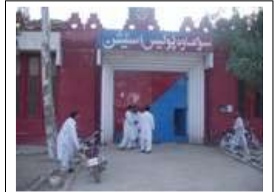
Fig 7: Picture of Sohawa Police Station
