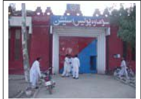
Fig 7: Picture of Sohawa Police Station
